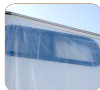
Plastic sheeting protects the sidewalls.
